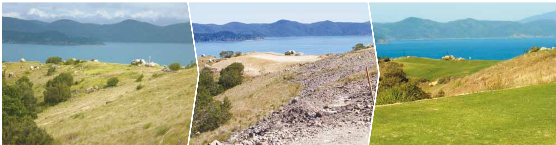
The three stages of construction for the 4th hole at Dent Island
